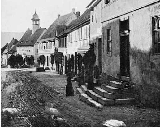
Fig. 12 Schultze-Naumburg, Paul: Street in Lobeda , 1909. Left picture: "Example of good curve design in a road. The configuration means that all of the house fronts are visible." Right picture: "Adverse road conditions. The road is not heading to any visible destination. The bend is hard and sharp."
